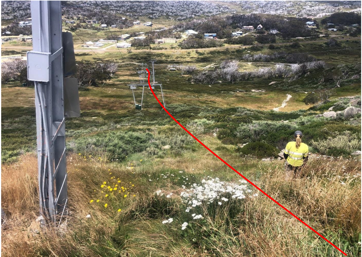
Photo 1: The replacement line will follow the alignment of the existing uphill line, with the exception of a deviation near the bottom to avoid two patches of Perisher Wallaby Grass.
